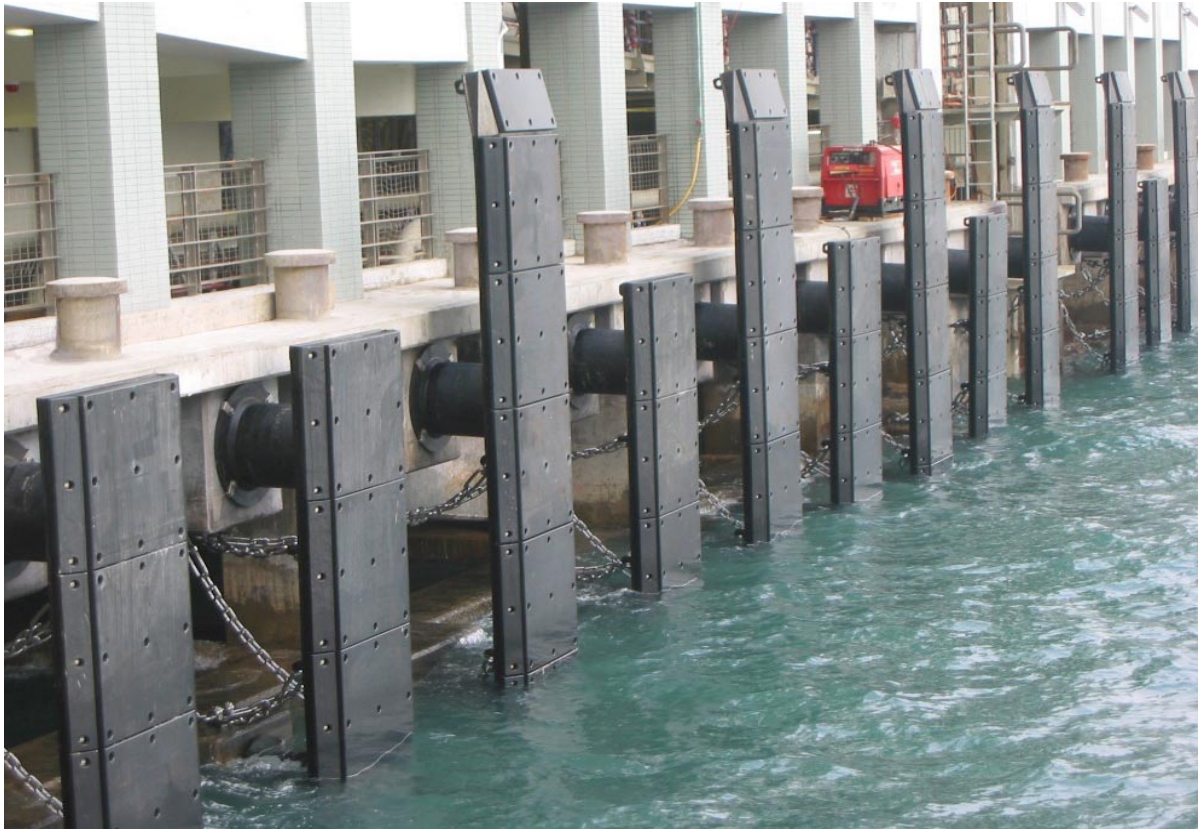
Plate 3 – Cell Fenders with Front Panel
