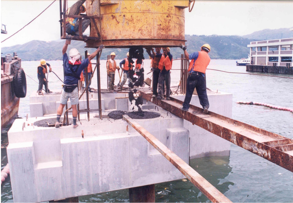
Plate 7 – Precast Concrete Pile Cap
