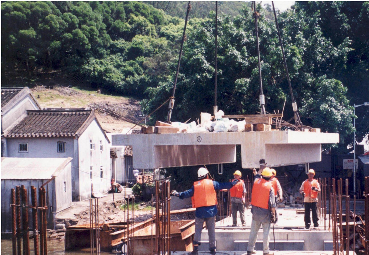
Plate 8 – Precast Concrete Beam and Slab
