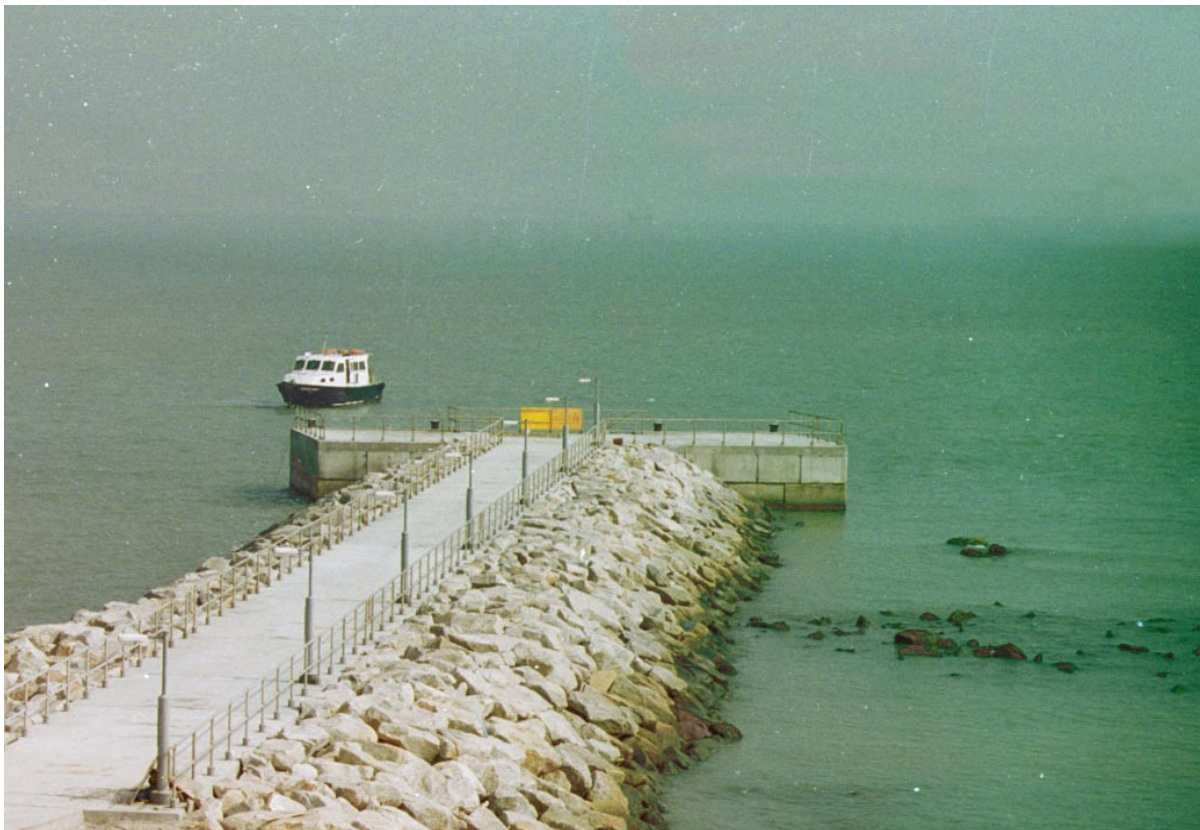
Plate 2 – Solid Pier made of Precast Concrete Blocks and Rubble Mound Catwalk
