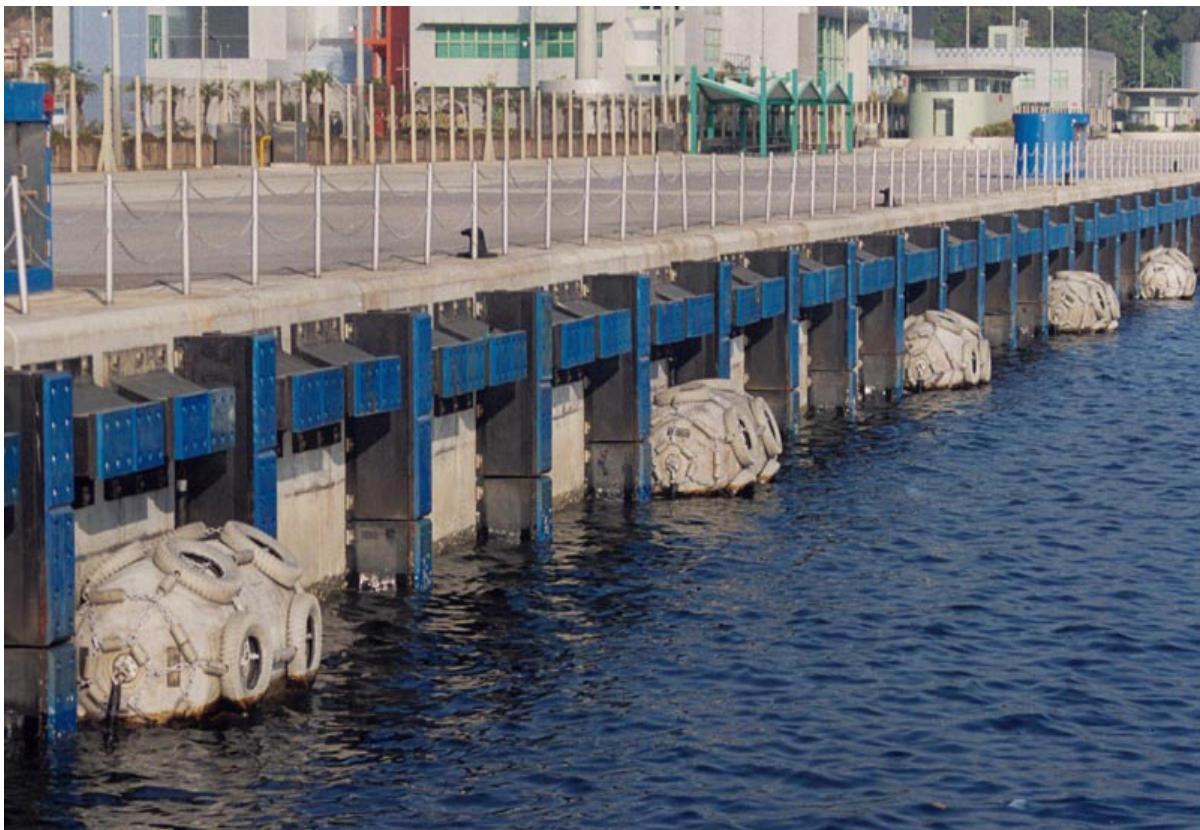
Plate 4 – Pneumatic Fenders and Arch Fenders
